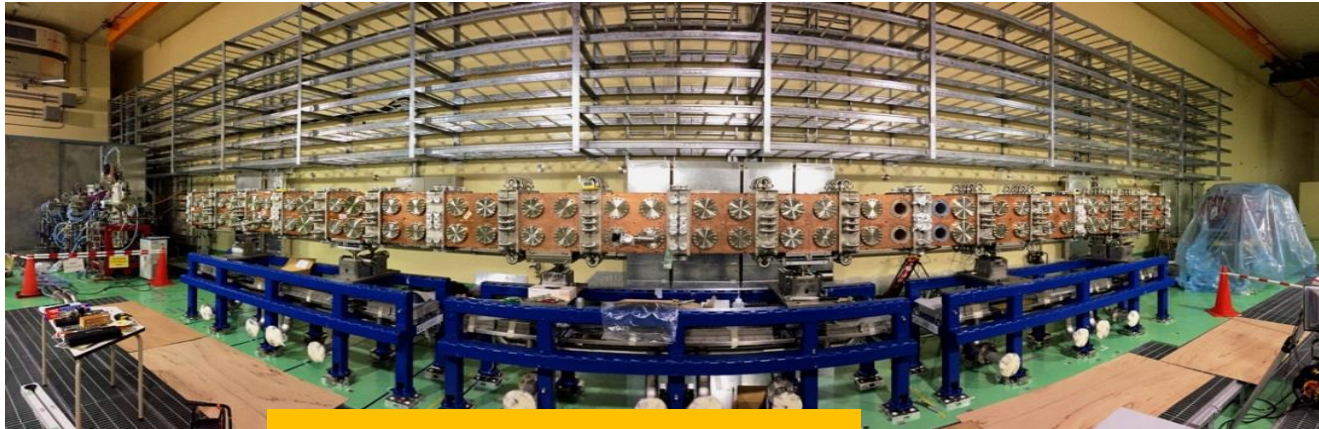
RFQ under commissioning
