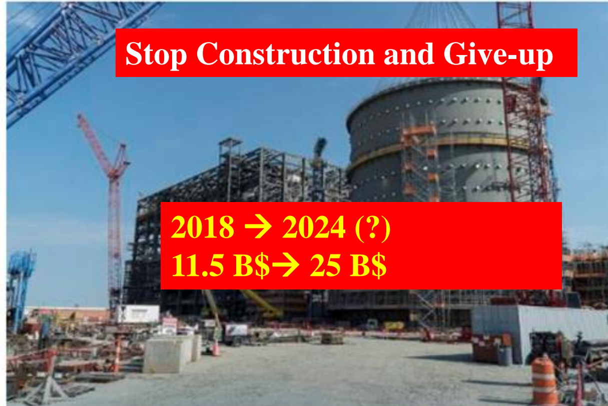
Summer unit 2, pictured on 9 June after placement of the unit's third and final containment ring (image: SCE&G)
