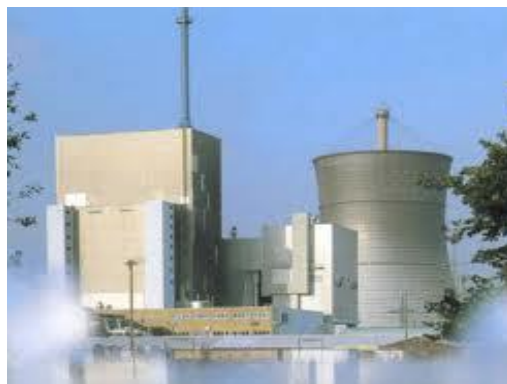
THTR, Germany 300 MWe 1986-89
