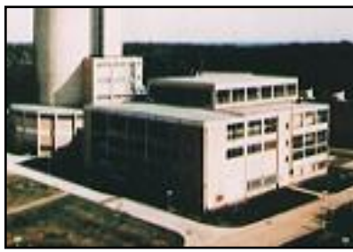
AVR, Germany 15 MWe 1967-88
